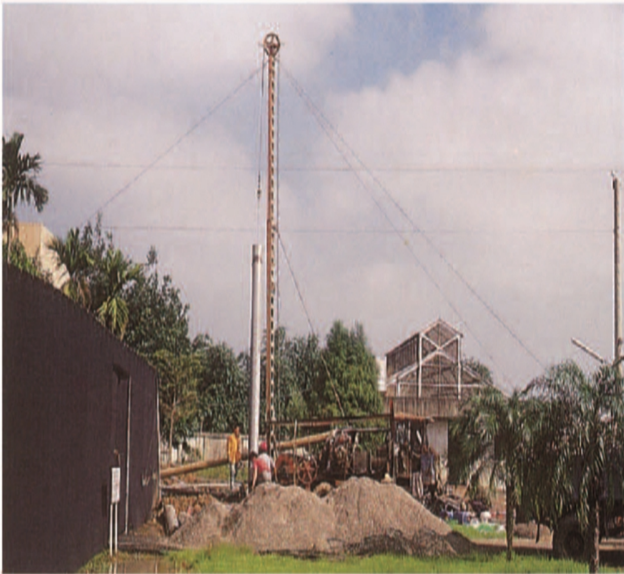
▲凿井工程 Well drilling engineering
