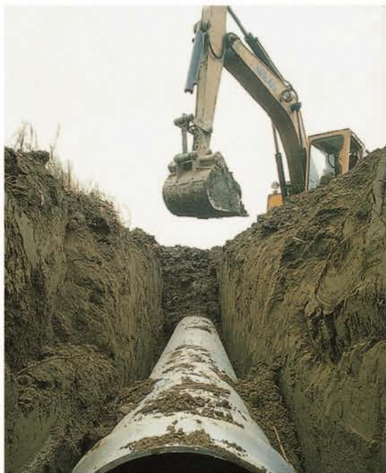
▲自来水工程 Water supply engineering
